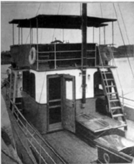
Aft portion of Georgiana III's deck cabin (The Motor Boat 1916)
